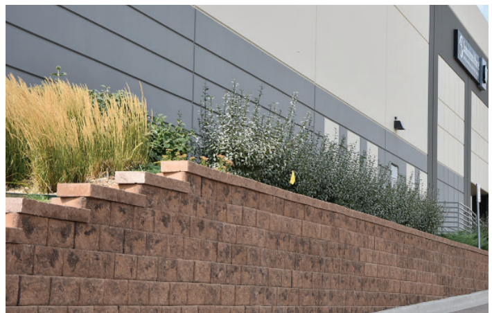
Example of approved retaining wall
