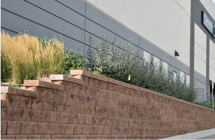
Example of approved retaining wall
